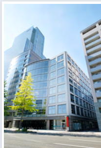
HF SENDAI ICHIBANCHO BUILDING
