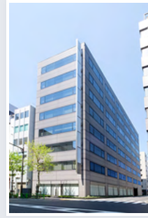
HF NIHONBASHI KABUTOCHO BUILDING
