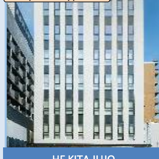
HF KITA JUJO BUILDING
